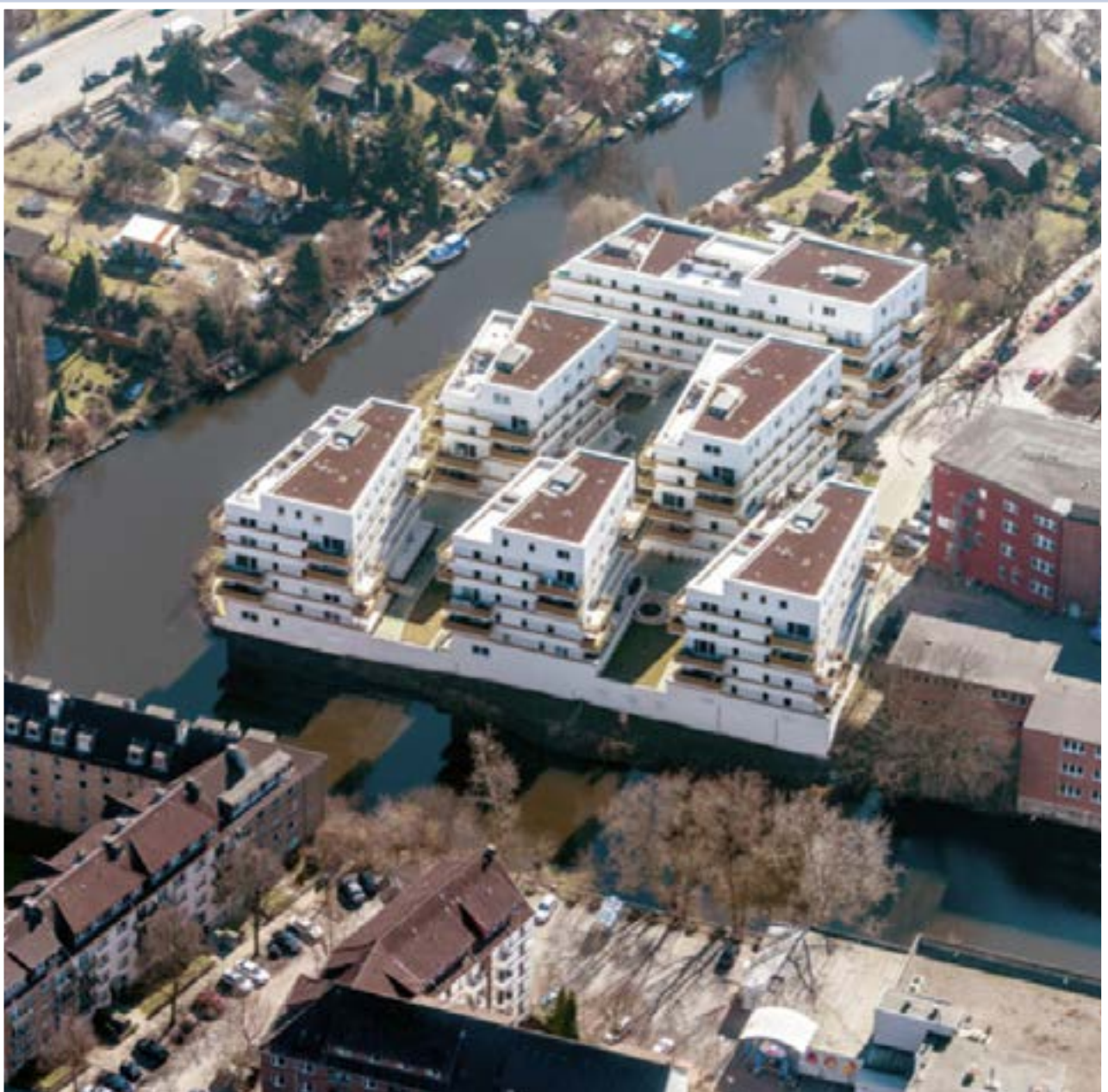
Hanseterrassen, Hamburg. Foto: Falcon Crest Air. www.falconcrest.com
